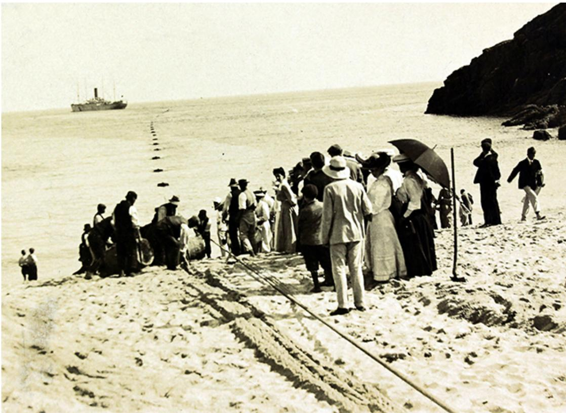
Fig. 1. *The cables ship Colonia lands a cable at Porthcurno in the United Kingdom, 1906, Photographer Unknown, Photograph, © Cable & Wireless Communications 2013. (By permission of Porthcurno Telegraph Museum.)*
