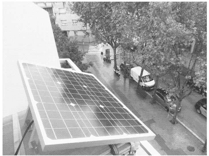
The 50W solar PV panel in our original configuration. Since January 2019, we have been running the website on solar panels of 10W and 30W.
